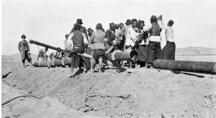
Figure 8. Laying oil pipelines from Masjed Soleiman to Abadan by local (Bakhtiari) laborers working for Anglo-Persian Oil Co., 1910
