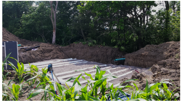
Figure 1.3. Example of a confined bed P removal structure. Downward flow.
