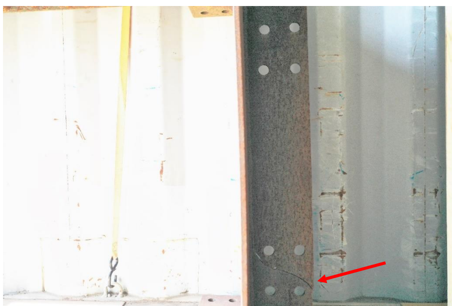
Figure 98 UAS inspection of steel elements, enhancing to see defects hidden by shadows.
