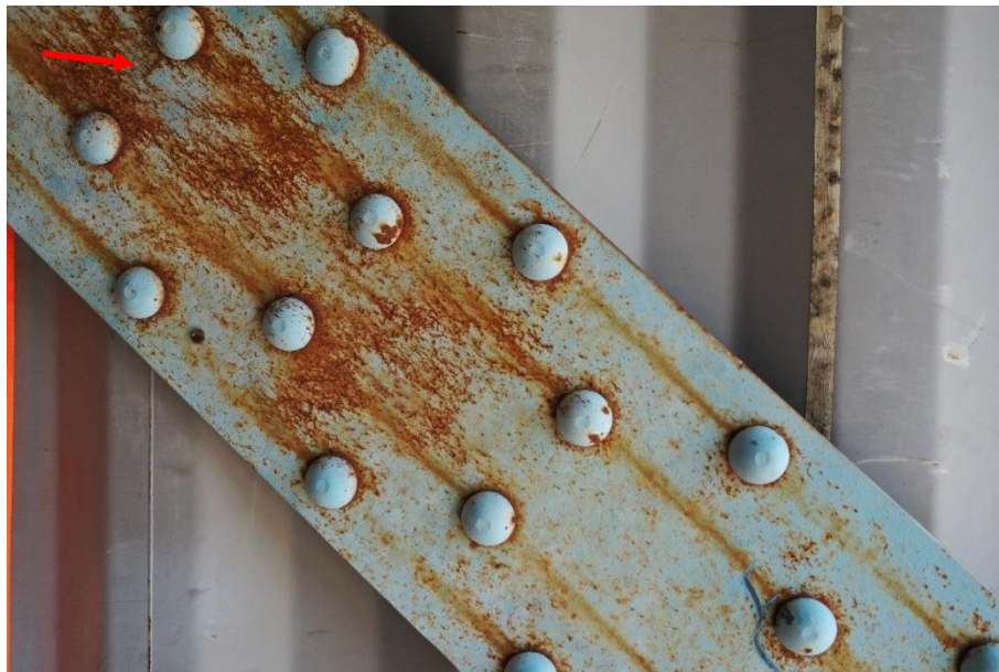
Figure 100 UAS inspection of steel elements.
