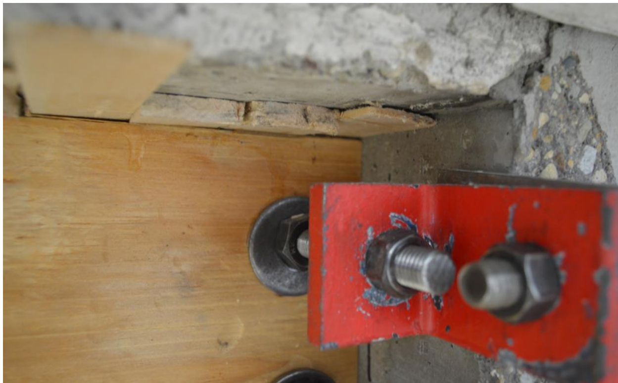
Figure A-13: Wood Shims Filling Frame to Infill Edge Gap
