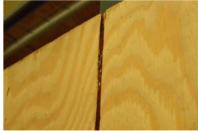
(b) Multi-ply face splitting
