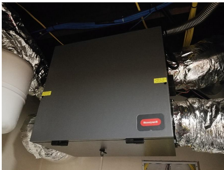
Figure 2.4 Energy recovery ventilator (ERV) in the basement of the ReNEWW House.
