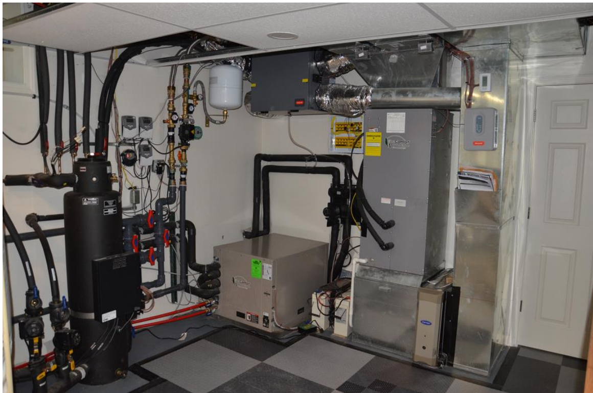
Figure 2.3 Air handling unit (AHU) in the basement of the ReNEWW House.
