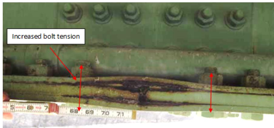
Fig. 5.1. Increase in the bolt tension due to bending of the splice plates
