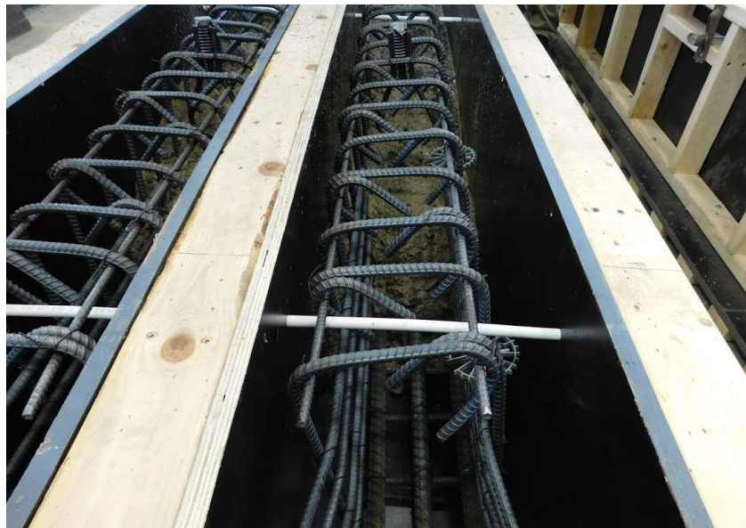
Figure 2.15: Reinforcing Cages Inside Forms
