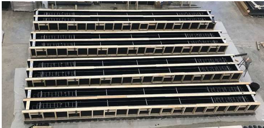
Figure 2.14: Completed Formwork
