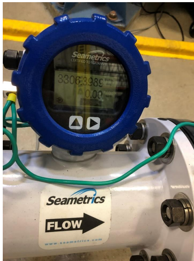
Figure 4.23: Magnetic Flowmeter
