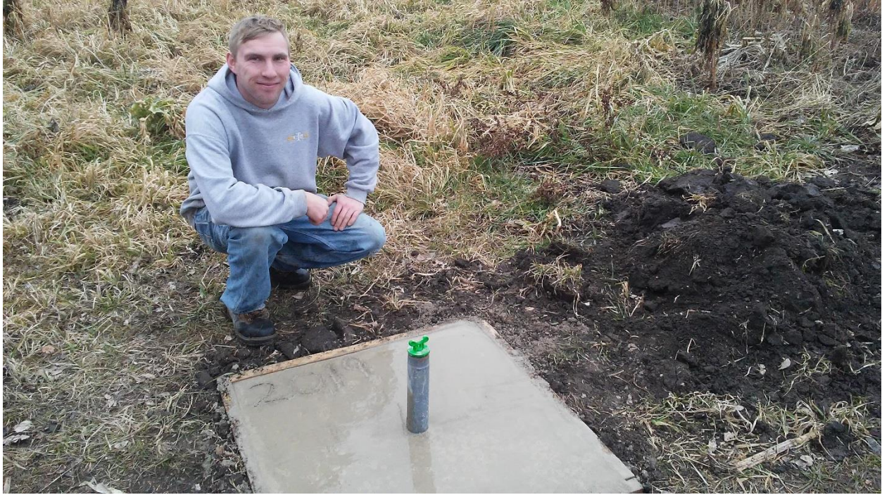
Figure 39 Concrete Pad at Test Well 2 (Personal photograph, 2019)
