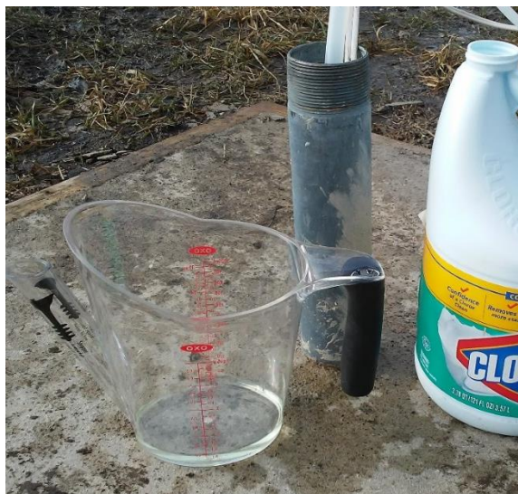
Figure 41 Disinfection of Test Well 2 (Personal photograph, 2019)
