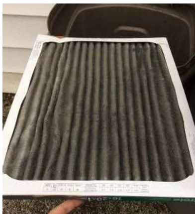
Figure 2.2 Dirty air filter to be replaced.
