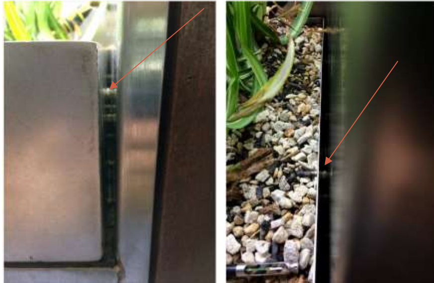
Figure 3.1 Initial air seal assessment revealed Growstone rocks between the plant trays and Biowall housing.
