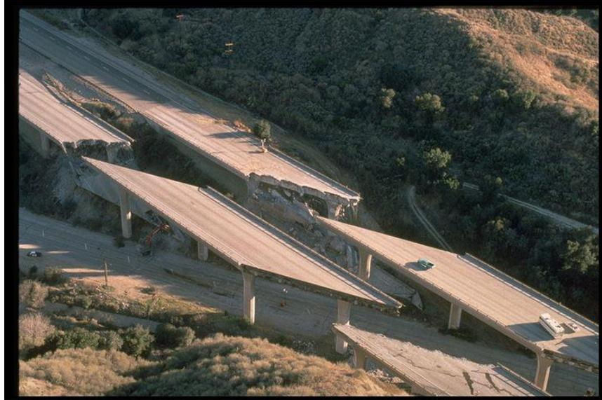
Figure 2-4: Bridge Failure Due to Unseating at Support During the 1994 Northridge California Earthquake (Sozen et al., 2005)
