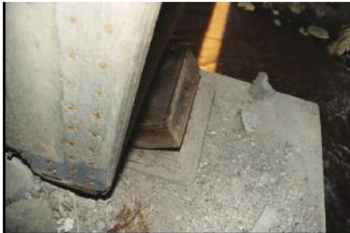
Figure 2-6: Failure of an Elastomeric Bearing Due to Excessive Longitudinal Displacement
