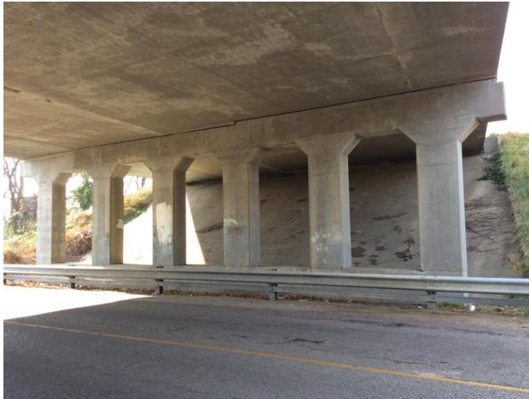
Figure 3-2: Multi-Column Bent Substructure (BIAS,2018)
