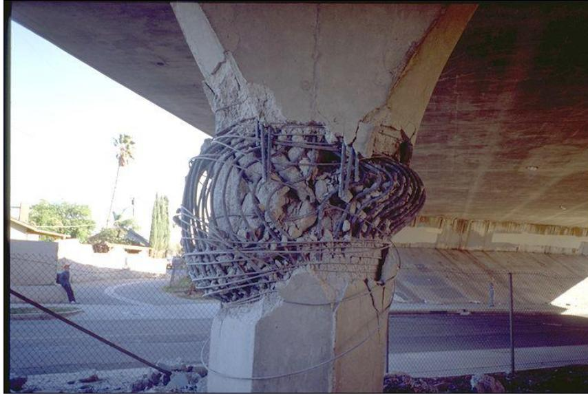
Figure 2-5: Column Failure of a Bridge During the 1994 Northridge California Earthquake
