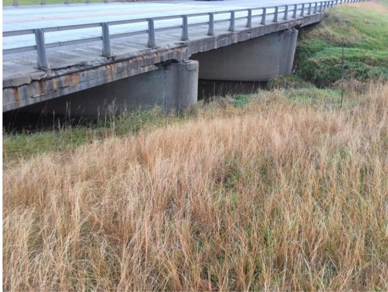
Figure 3-3: Wall Type Substructure (BIAS, 2018)
