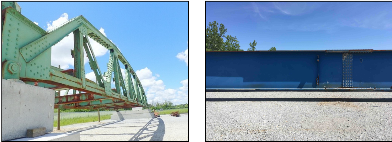
Figure 5.13. : Bridge components at Purdue’s S-BRITE Bridge Component Gallery [113]. Left: Indian Trail Road Bridge (91-ft. Pony Truss); right: Virginia Avenue Bridge (155-ft. Main Span Girder Bridge).
