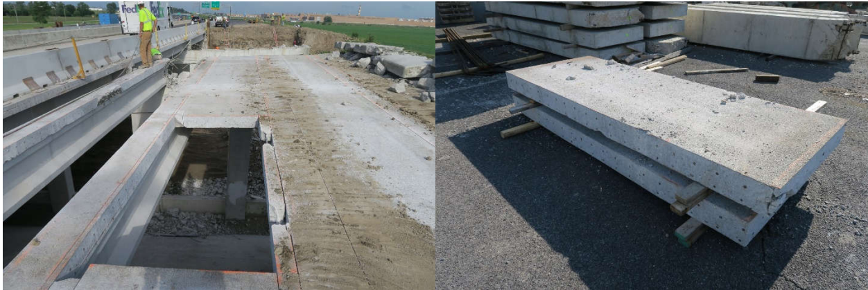
Figure 3-3. Original Deck Sections Removed from I-469
