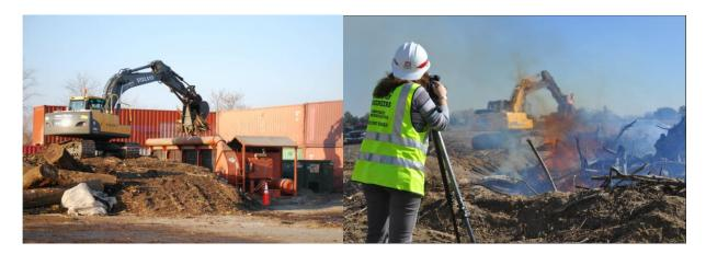
Figure 2-7 Air curtain incinerator (left) and open burning system (right) *Photo credit: Clay Church and Billy Birdwell / USACE*
