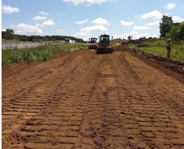
Figure 7.5 Subgrade compaction for No. 30 backfill soil using vibratory compactor for the construction of ramp at US 20 and IN 2 intersection at Rolling Prairie, IN
