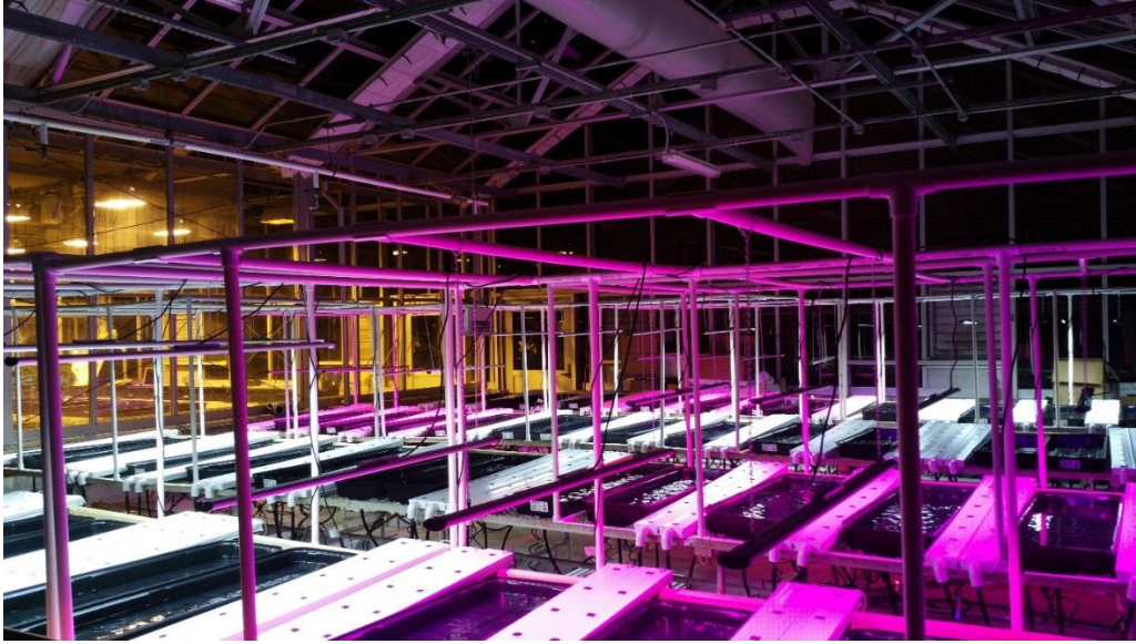
Figure 2.1: Image of supplemental lighting and their PVC supports in the greenhouse
