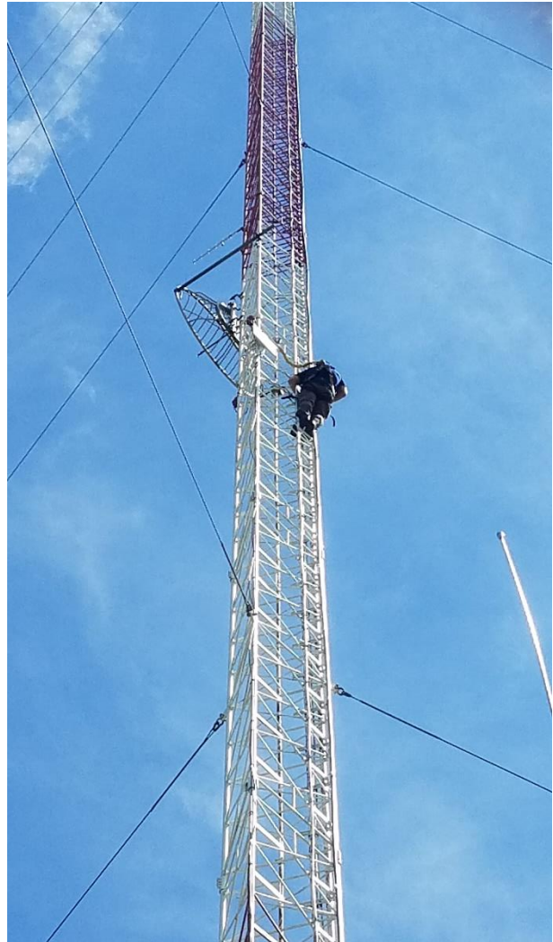
Figure 3.6: Installation of the Access Point
