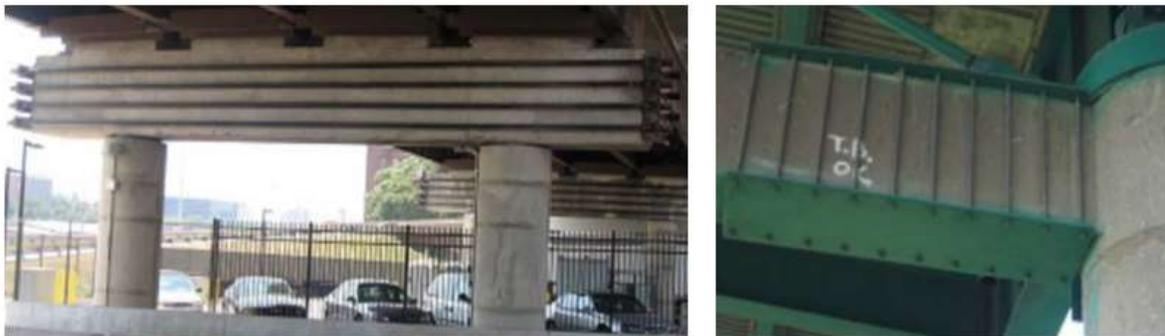
Figure 2-8. External Post-Tensioning (left) and Shear Reinforcement (right) for Bent Cap Strengthening (Timothy et al., 2011)
