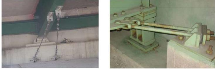
Figure 2-6. Restrainer Cables (Left) and Restrainer Bars (Right) (Timothy et al., 2011)
