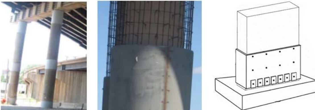
Figure 2-7. Steel Jackets (Left), RC Jacket (Middle), and Steel Plate Encasement with Steel Anchors (Right) (Timothy et al., 2011; Timothy et al., 2011; FHWA, 2006)
