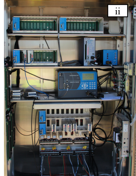
(b) Cabinet with controller and communication devices
