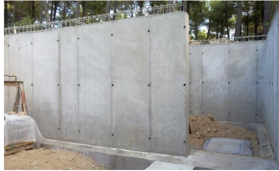
Figure 3.9. Wall poured until slab bottom
