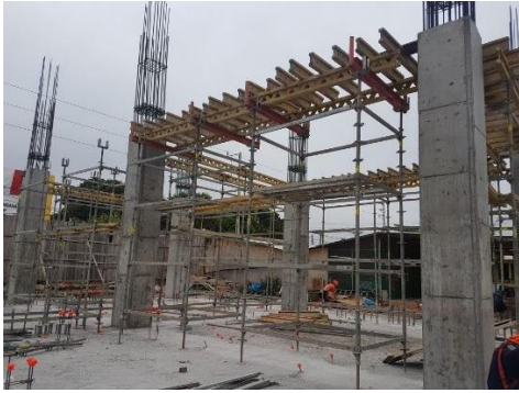
Figure 3.8. Column poured until beam bottom
