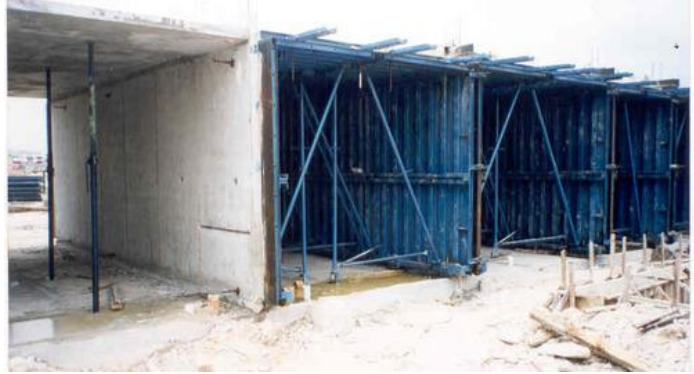
Figure 3.21. Monolithic structure with tunnel formwork
