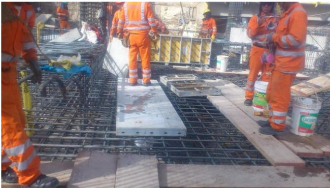
Figure 2.9. Formwork element used as a work platform
