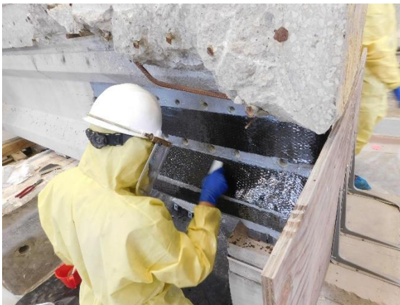
(e) Removing Excess Epoxy with Squeegee
