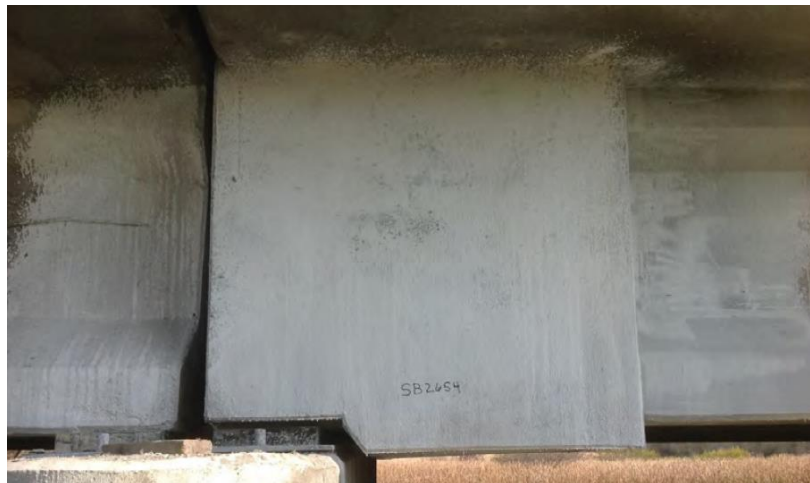
(b) Complete Shotcrete Repair
