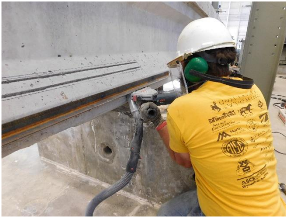
(a) Cutting NSM Groove
