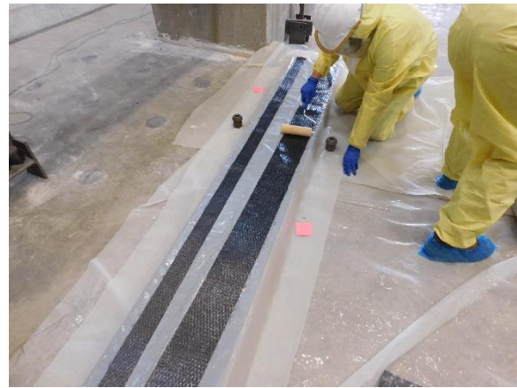
(b) Saturating Longitudinal FRP Strips
