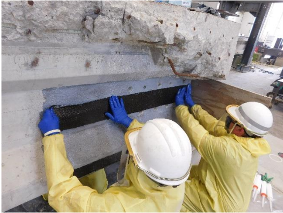
(c) Placing Longitudinal Strips
