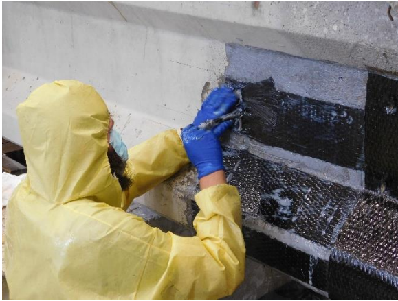
(c) Inserting Spike Anchor
