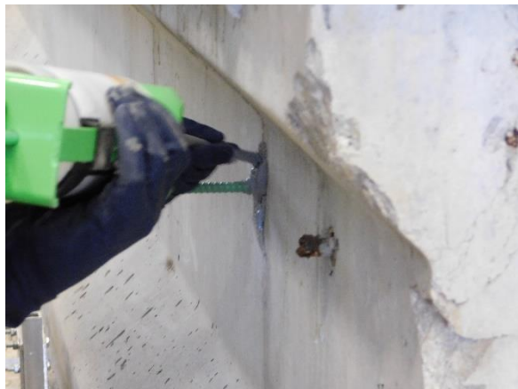
(h) Injecting Additional Epoxy
