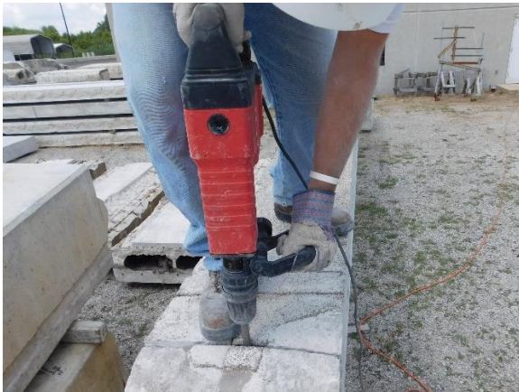
(c) Removing Concrete to Create Rectangular Repair Area
