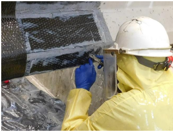
(a) Separating Fibers with Razor Blade
