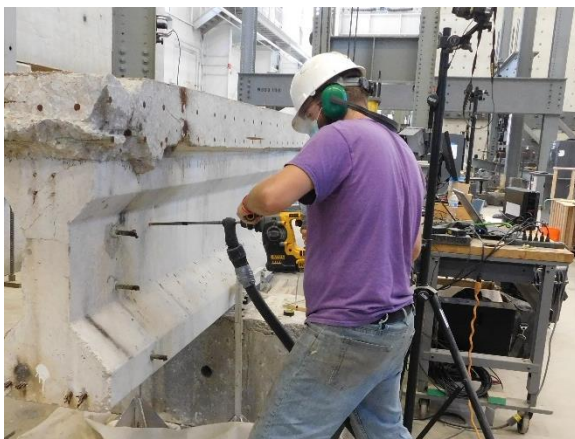
(a) Drilling Holes for No. 3 Bars
