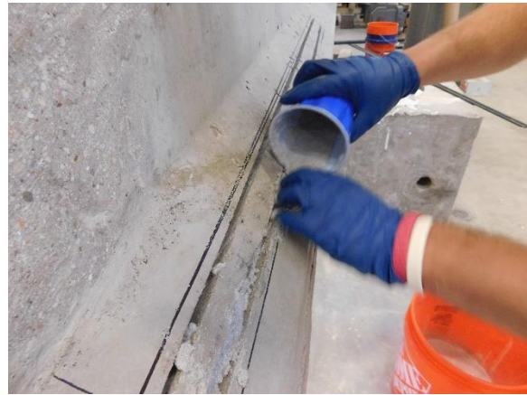
(b) Filling Groove with Epoxy Grout
