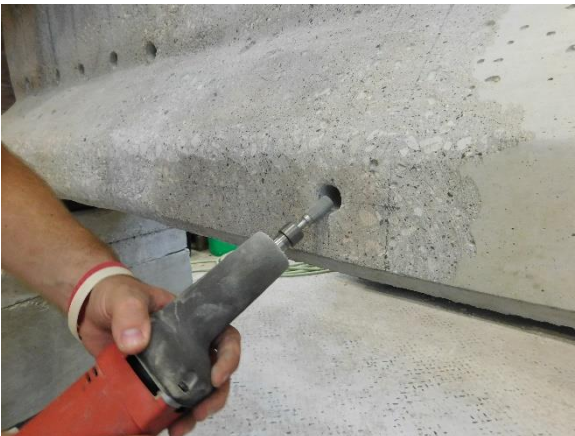
(g) Rounding Edges of Anchor Holes
