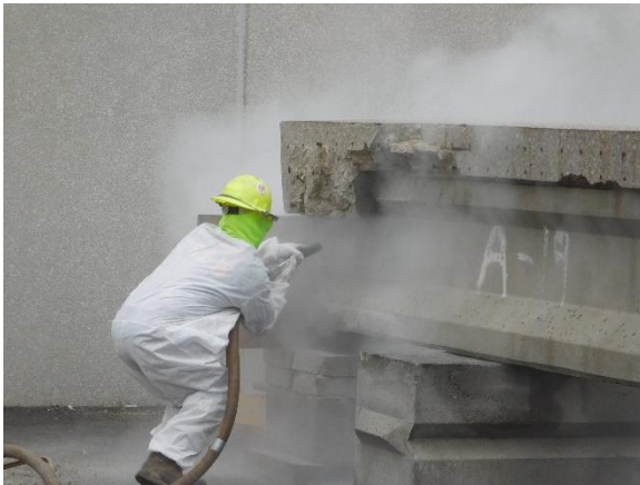
(e) Sandblasting for FRP Application
