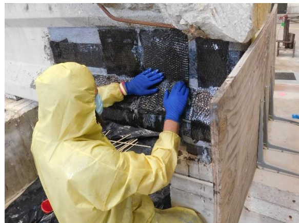
(h) Placing Patch Sheets
