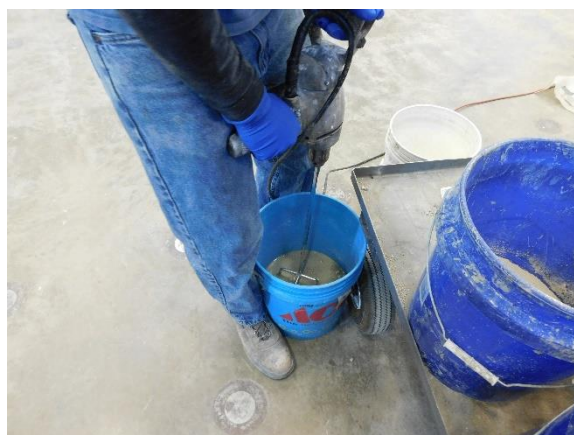
(b) Mixing Mortar
