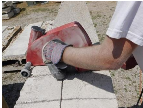
(b) Sawing Concrete Deck
