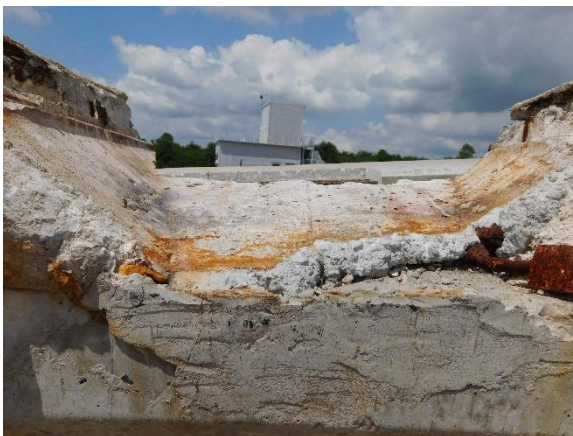
(a) Void Left After Drain Removal
