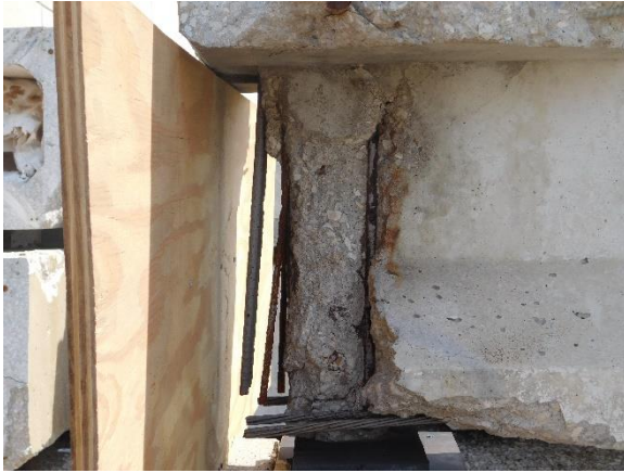
(c) Condition After Sandblasting
