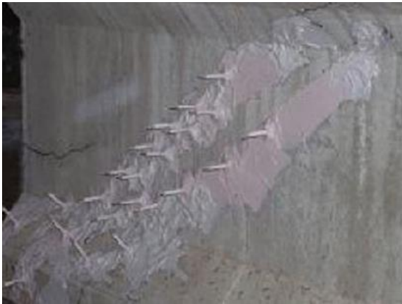
(c) Epoxy-Injected Cracks
