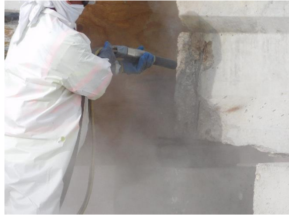
(b) Sandblasting to Remove Corrosion
