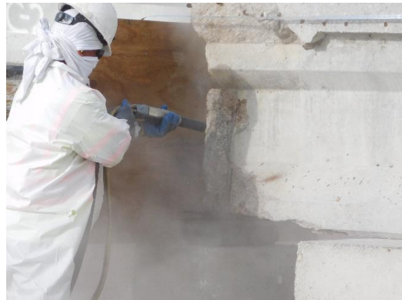
(b) Sandblasting to Remove Corrosion
