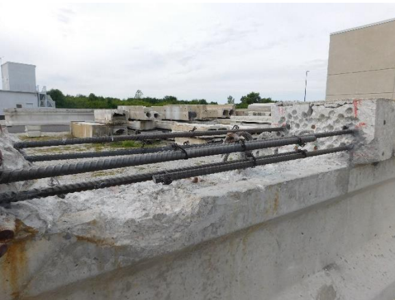
(c) Longitudinal Reinforcement After Placement
