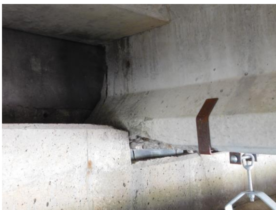
(a) Bottom Flange Deterioration
