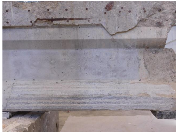
(e) Completed NSM Repair System
