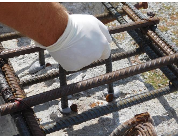
(e) Installing U-Shaped Bars
