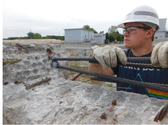
(b) Inserting Longitudinal Reinforcement
