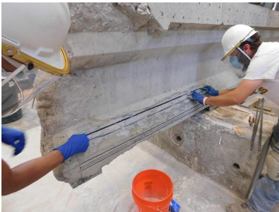
(c) Inserting NSM Strip
