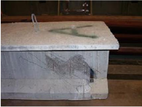
(a) Delaminated Concrete Removed
