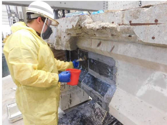
(f) Saturating Anchors
