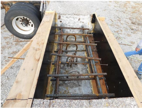
(a) Erected Formwork
