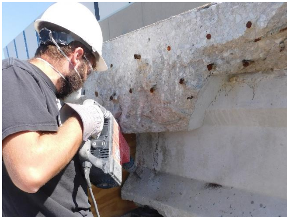
(a) Removing Delaminated Concrete
