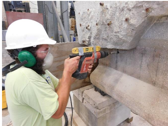
(f) Drilling Anchor Holes
