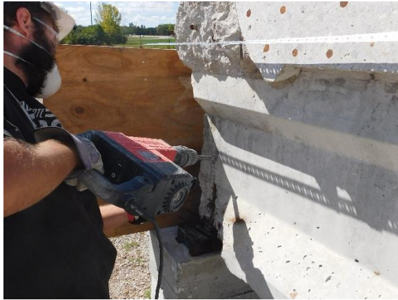
(a) Removing Delaminated Concrete
