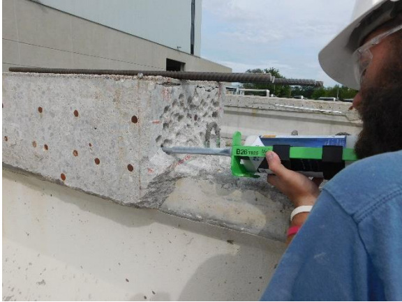
(a) Dispensing Epoxy for Anchorage of Longitudinal Reinforcement
