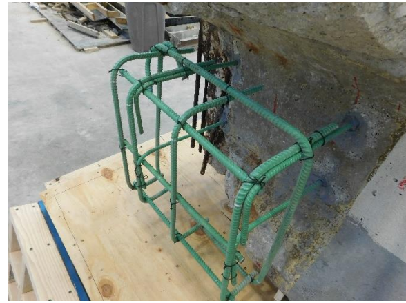
(l) Completed Reinforcing Cage
