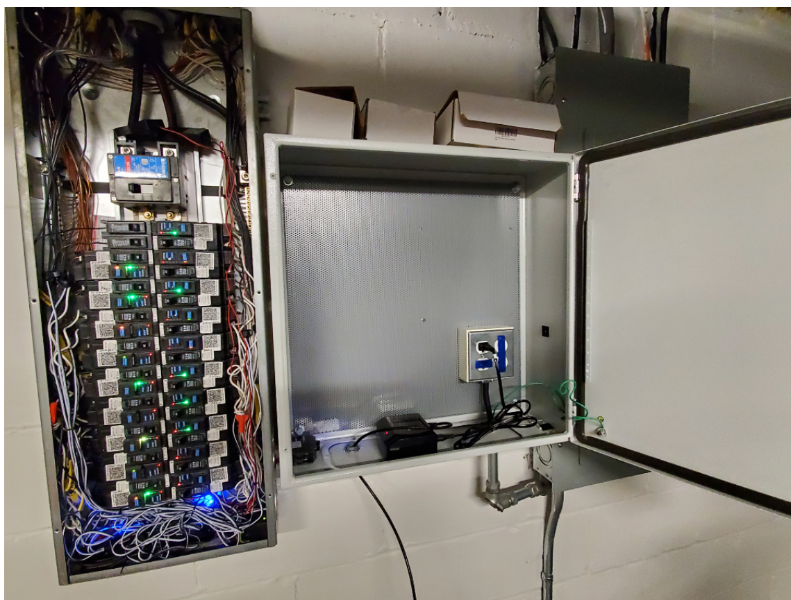
Figure 2.29. AC Load Center #1 TED Pro Home installation.
