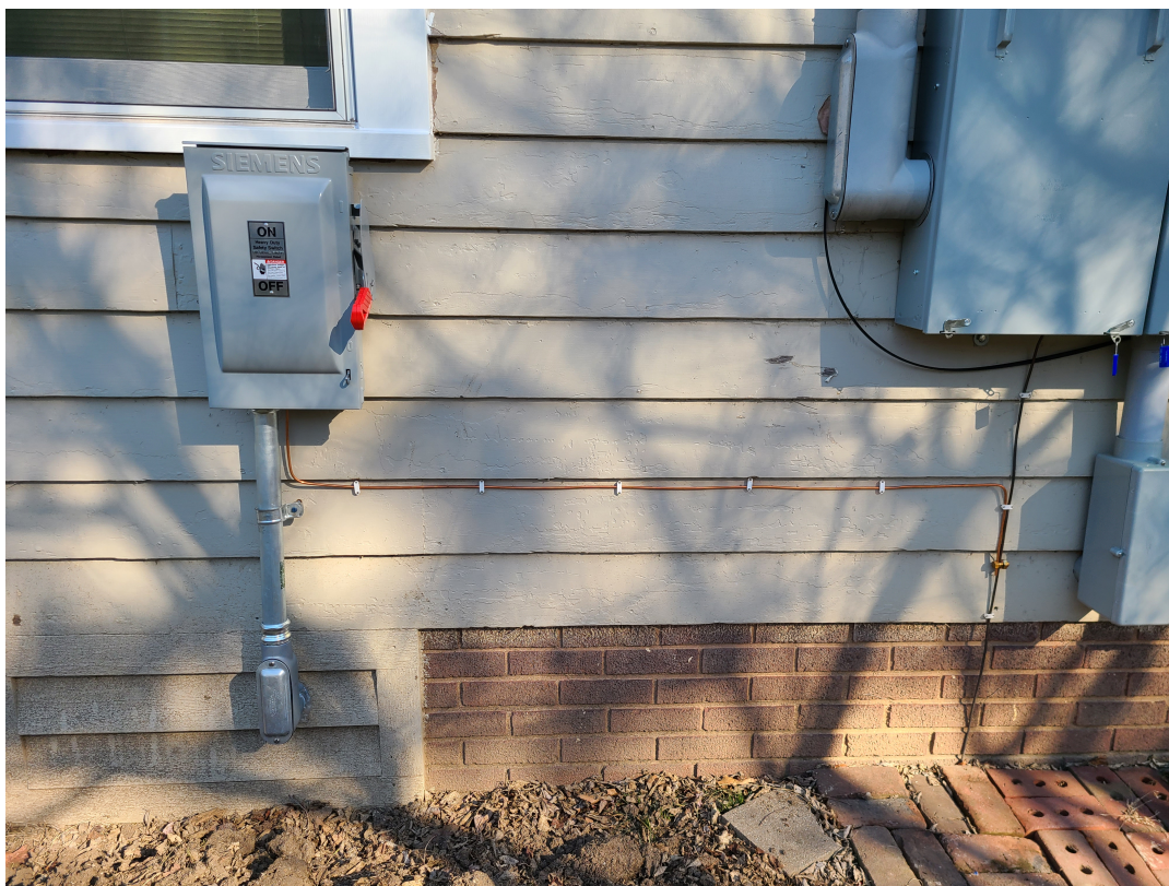
Figure 4.18. Nanogrid AC input utility disconnect location.
