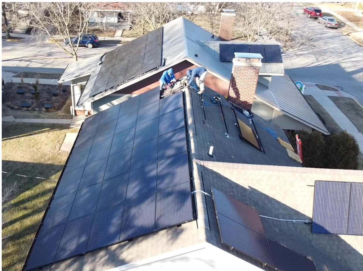
Figure 4.12. In-progress installation of the 14.3kW solar array.
