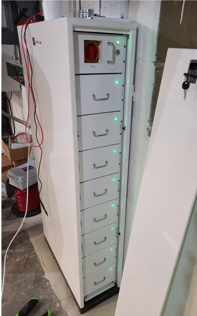
Figure 4.15. Installation of the 20 kWh battery system.
