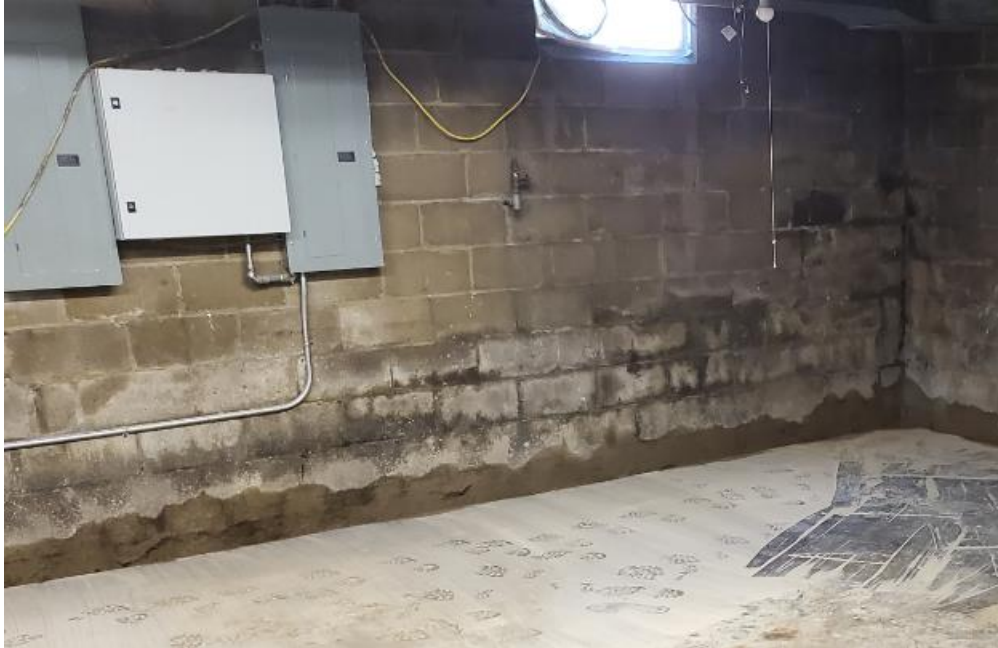
Figure 2.4. Presence of efflorescence on basement walls before waterproofing.
