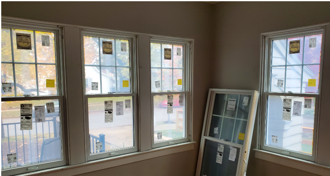
Figure 2.15. DC Nanogrid House Pella window installation.
