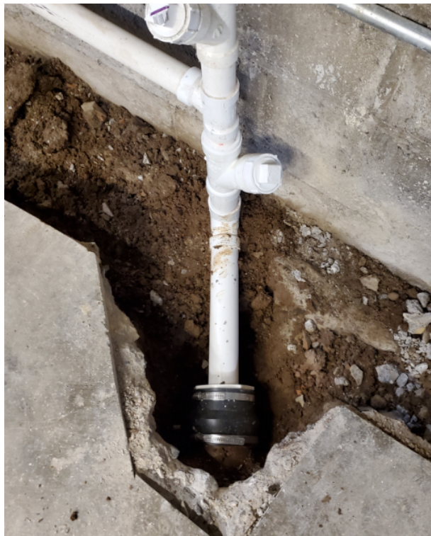
Figure 2.6. Drainage pipe after repairs.
