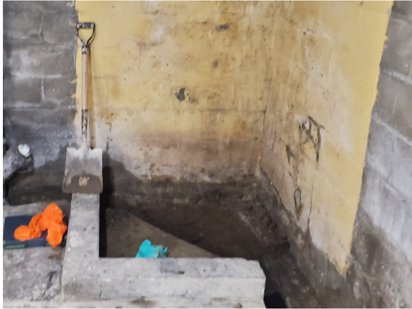
Figure 2.7. Excavation of foundation for sump pump and drain system installation.
