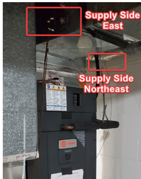
Figure 2.38. Thermocouple instrumented locations on the supply (east) side of the indoor unit.
