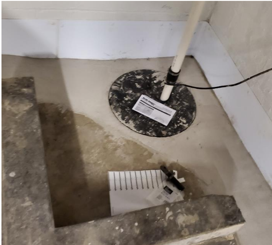
Figure 2.8. Completed installation of the sump pump.
