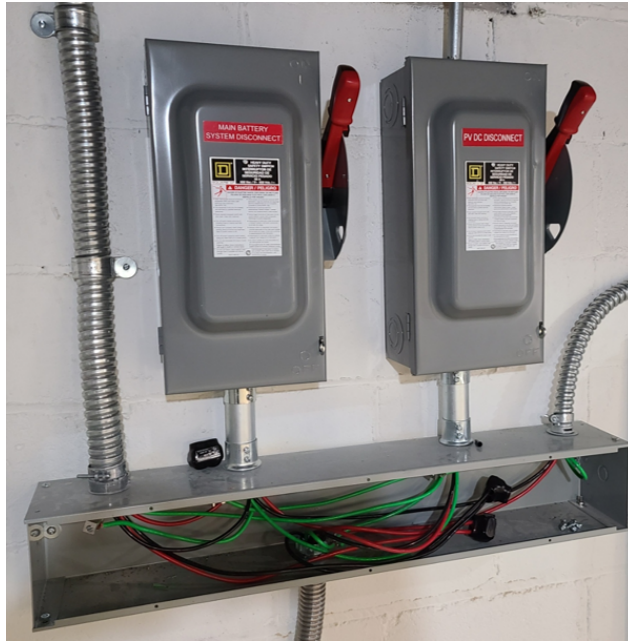
Figure 4.21. Solar PV and battery indoor disconnect locations.
