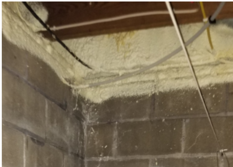
Figure 2.11. Basement spray foam installation.
