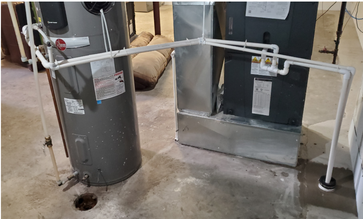
Figure 2.10. Completed condensation drainage line installation.
