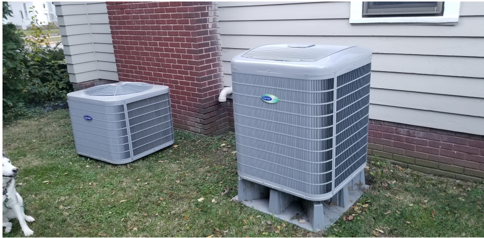
Figure 2.31. Carrier Greenspeed outdoor single and variable-speed heat pump unit comparison.
