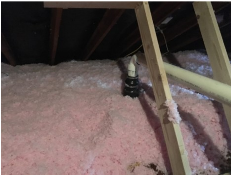
Figure 2.14. DC House attic after installing R-60 fiberglass blown-in insulation.
