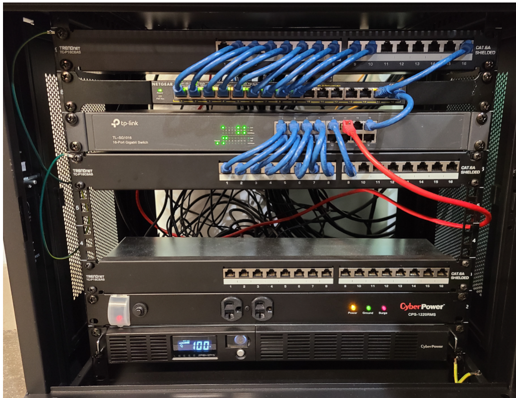
Figure 5.35. Networking server rack internals.
