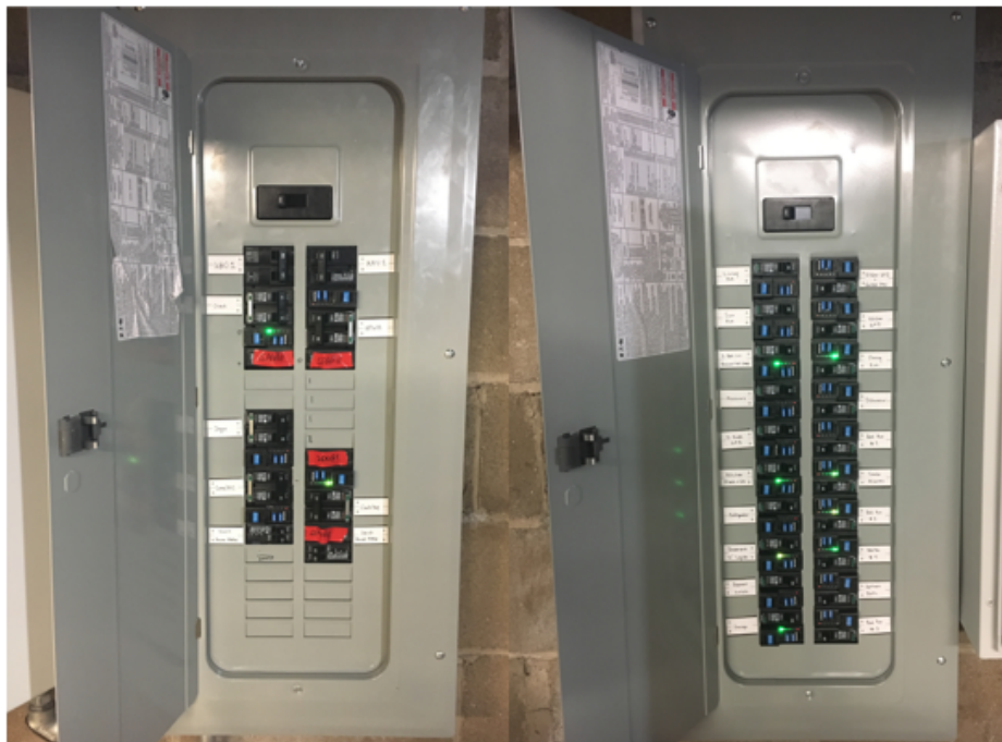
Figure 2.24. AC load panels after EMCB installation.
