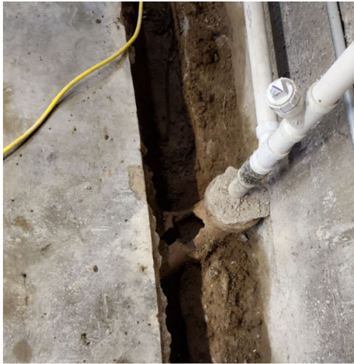
Figure 2.5. Cracked ceramic drainage pipes.
