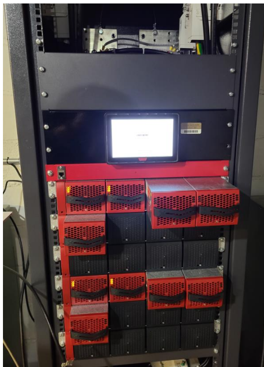
Figure 4.28. Commissioning of the bidirectional Sierra inverter system and modular Bravo ECI components.
