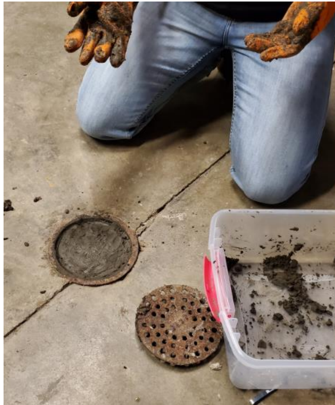
Figure 2.9. Sealed sewer line access with hydraulic cement.
