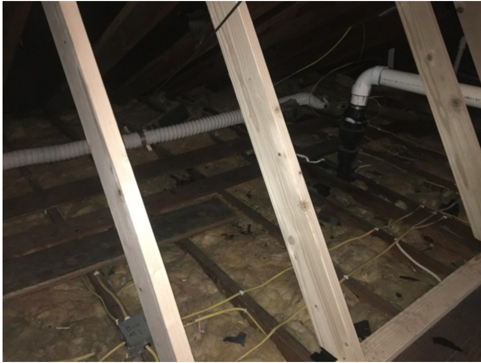
Figure 2.13. DC House attic with less than R-20 insulation.
