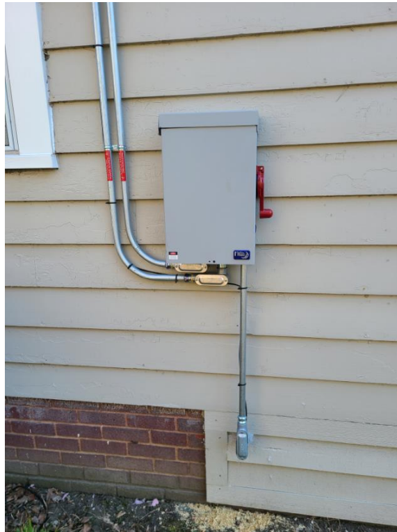
Figure 4.19. Solar PV combiner and disconnect location.
