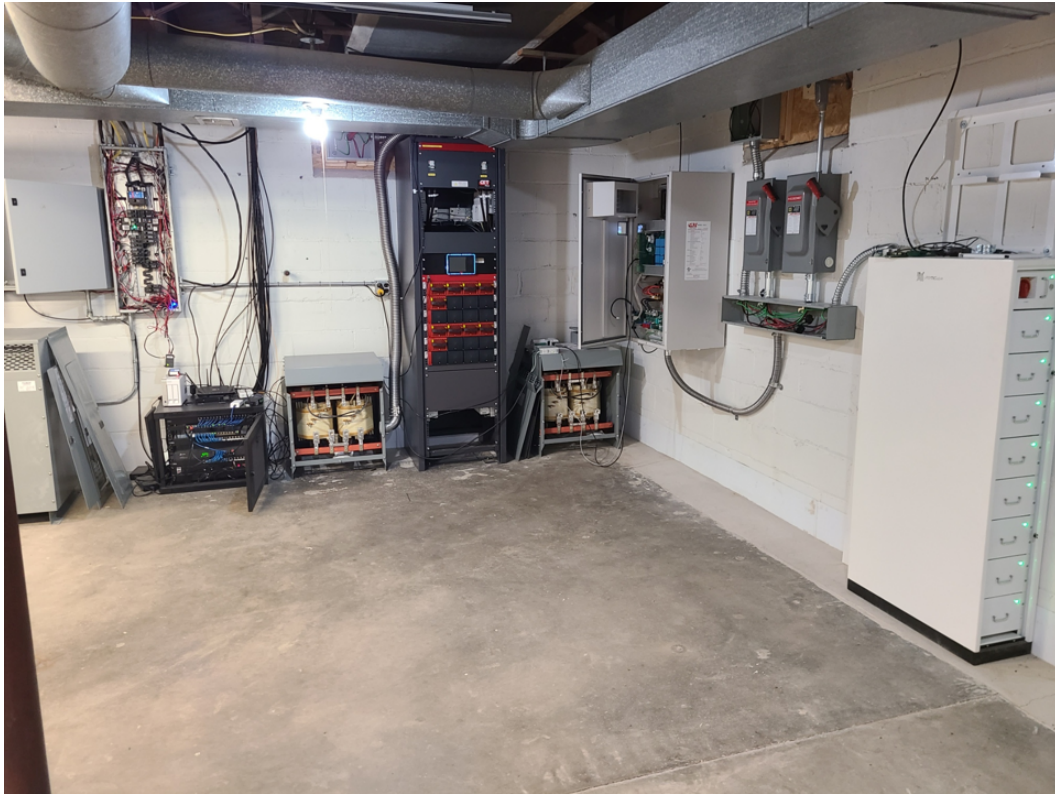
Figure 4.26. Assembled and installed DC nanogrid equipment.
