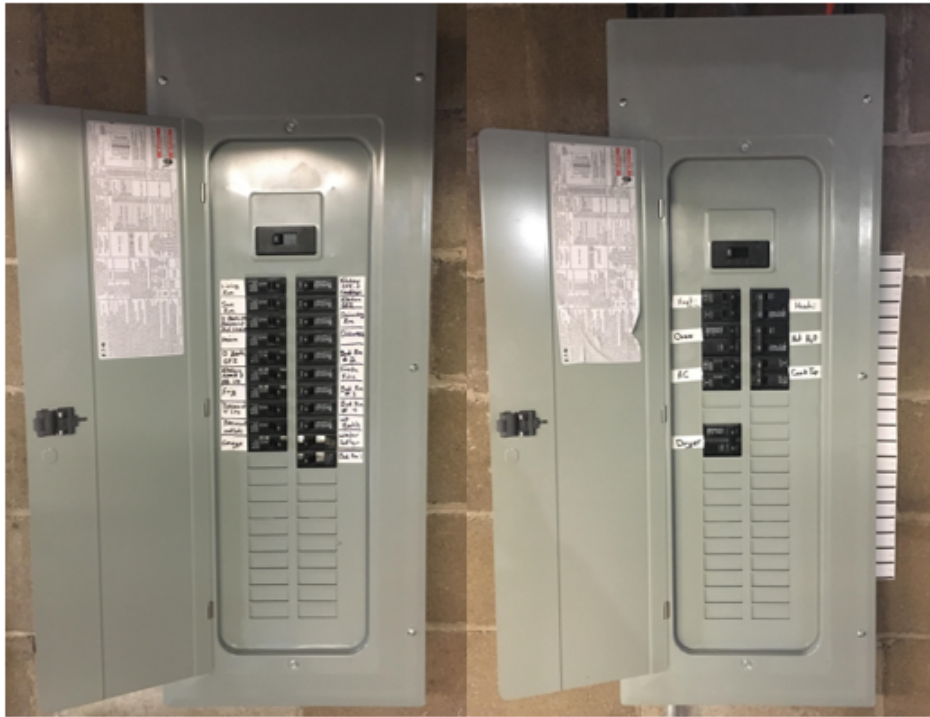
Figure 2.23. AC load panels before modifications.
