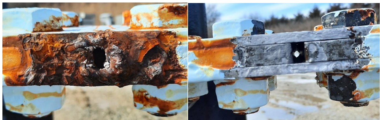
Figure 4.19. Surface and gap condition before and after pressure washing the connection.
