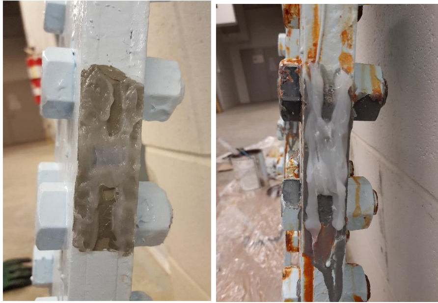
Figure 4.22. Caulk application for initial and repair conditions.
