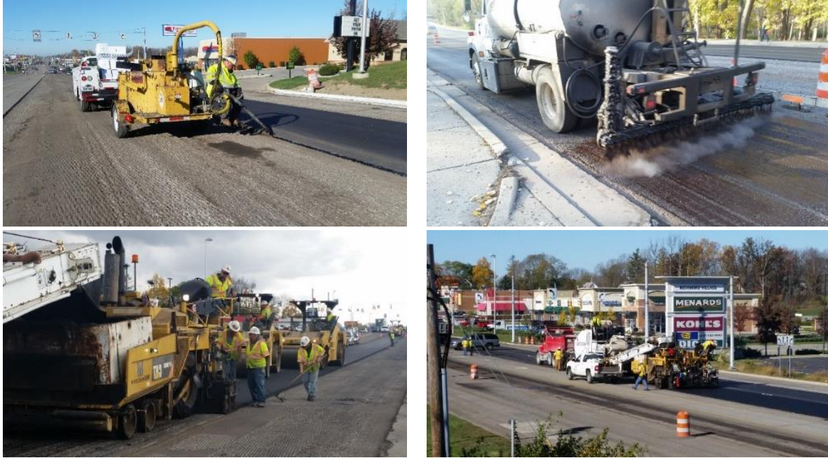
Figure 5.5. Asphalt mixture placement.
