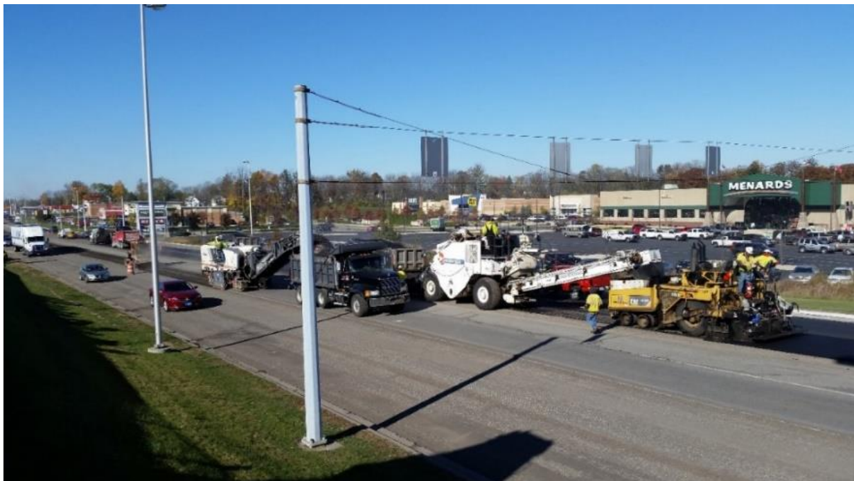
Figure 5.1. Milling and paving operations on US 40 in Richmond, Indiana.
