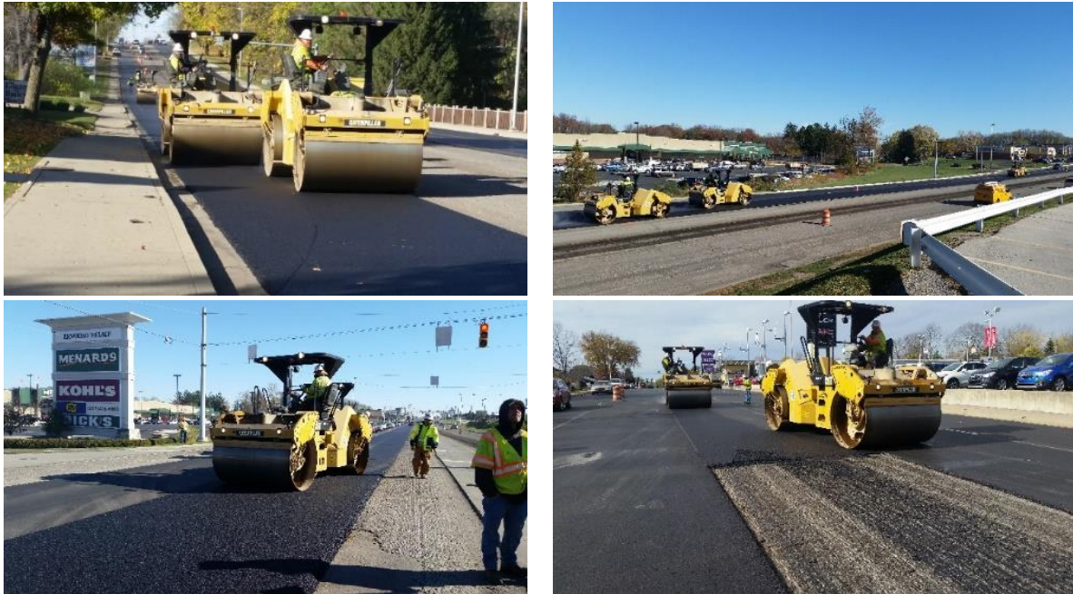
Figure 5.6. Mixture compaction.
