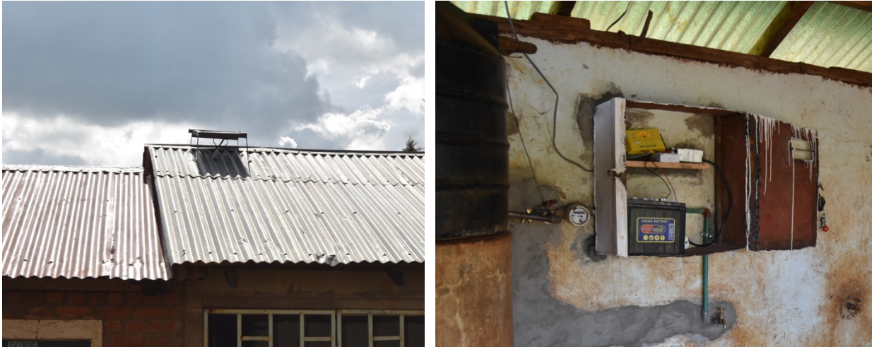
Figure 7.5. System components that were designed and constructed by the welder; (a) a solar panel bracket to hold the panel in place on the roof and locks so the panel cannot be stolen, and (b) a box to protect the system from tampering.
