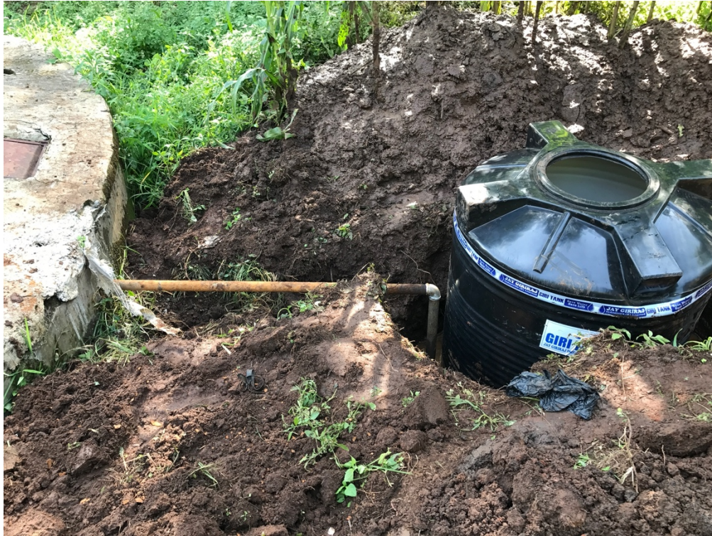
Figure 7.3. Standard sand filter that was installed after the source water (spring) and before a storage cistern from which water is pumped to schools A and B. School C received their own filter of the same design
