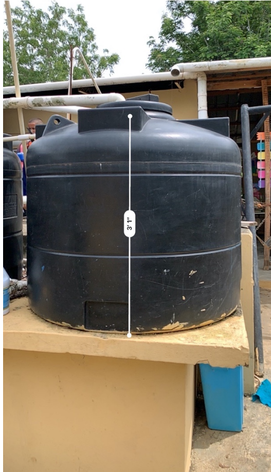
Figure 6.3. Elevated tinaco used to store treated water so that it can be gravity fed to drinking water taps and handwashing stations.
