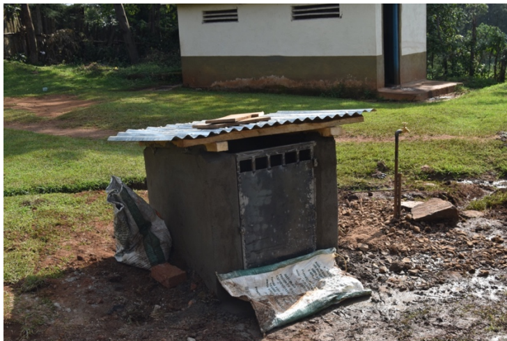
Figure 7.6. Structure built by a local mason to support and protect the water treatment system at school B because their tap was free-standing in an open field.
