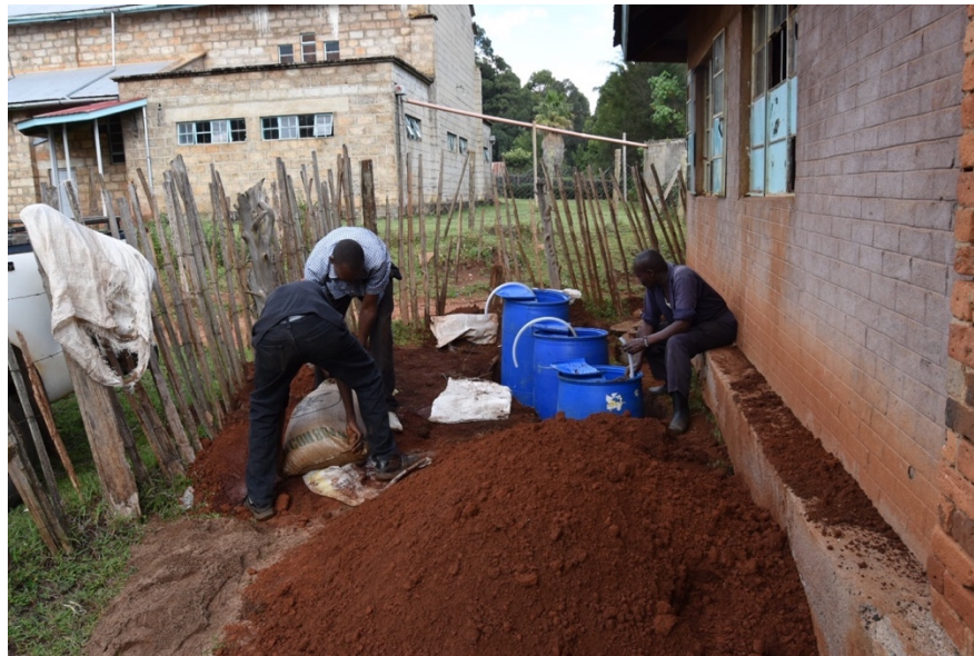
Figure 7.1. Initial installation of a series of slow-sand filters installed behind one of the classroom buildings at school A.
