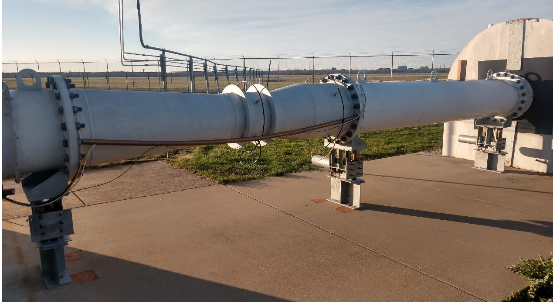
Figure 2.4. Outdoor inlet section with addition of constant-spring support legs.
