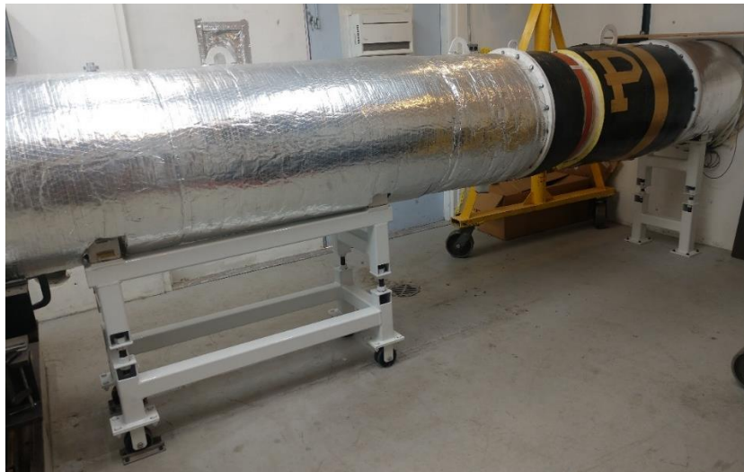
Figure 2.5. Adjustable leg supports for indoor inlet ducting and rubber transition for thermal growth in axial direction.
