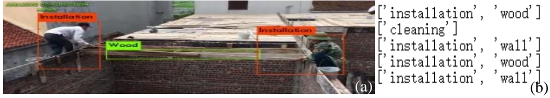
Figure 37. (a): Successful detection of installation action with associated wood object, (b): An example of post processing labels.
