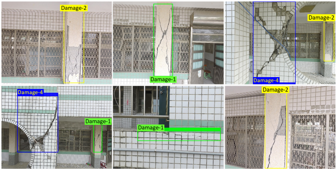
Figure 2.11. Damage detection results for images captured by a UAV post Taiwan earthquake (2016). Predicted boxes for Damage-1 (surface crack), Damage-2 (spalling), Damage-3 (spalling with exposed rebars), and Damage-4 (severely buckled rebars) are shown in different colors.
