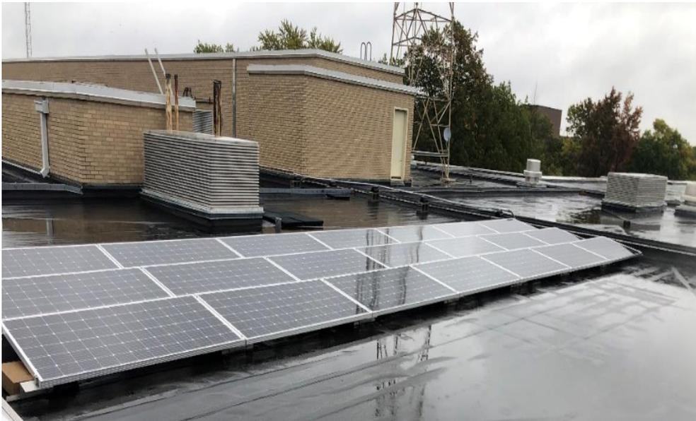
Figure 6.3: 7.6 kWp PV array mounted on the Kettler Hall rooftop at Purdue University Fort Wayne campus.
