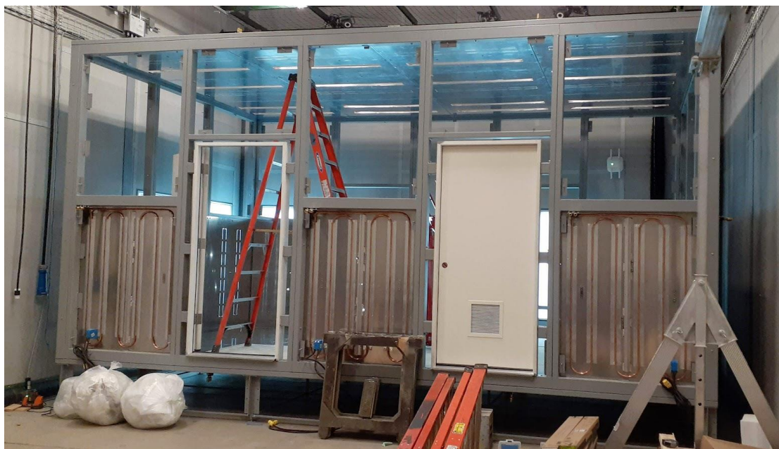
Figure 4.11 HBIL installation day 2 - full frame assembled
