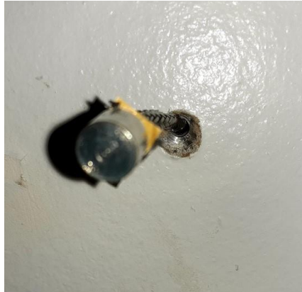
(b) Drywall hole to embed cylindrical head
