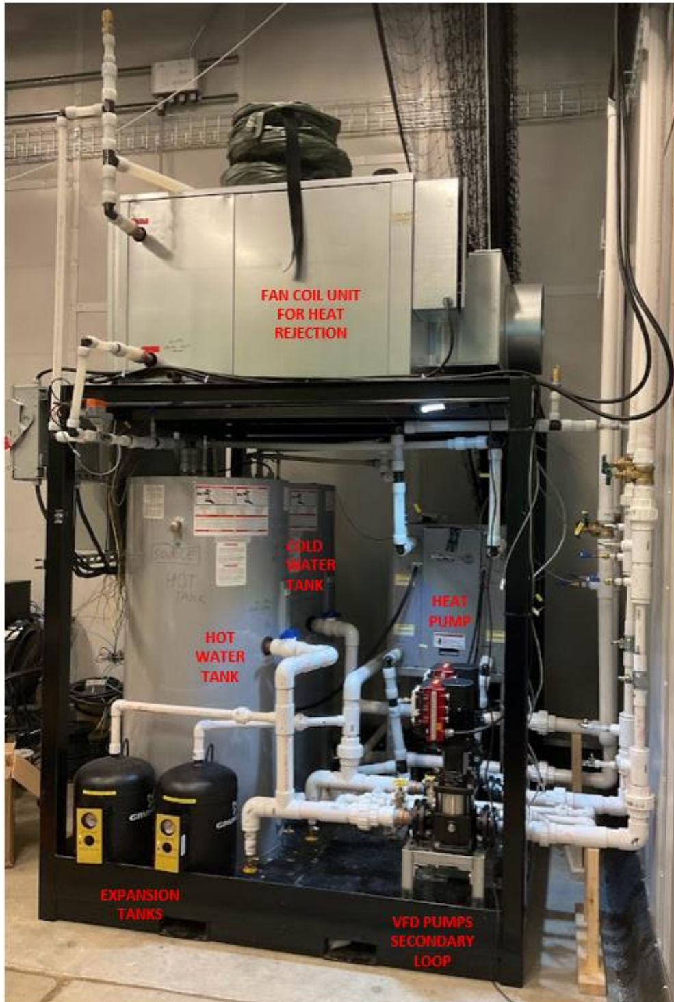
Figure 4.19 HBIL-primary loop equipment skid
