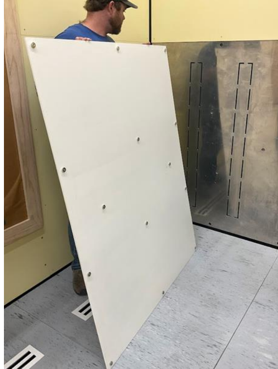
Figure 4.8 HBIL interior surface treatment panel removed at Bridgewater Studio
