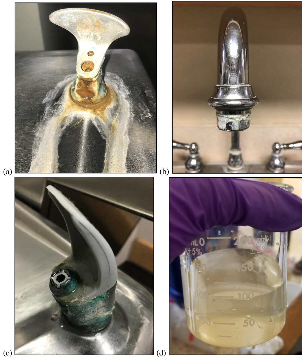
Figure 2-3. Fixture conditions at (a) Building A, (b) Building C, (c) Building D, and colored water from (d) Building D in March 2020. A drinking water fountain from building A has been changed with new drinking water fountain with filters after buildings re-opened.
